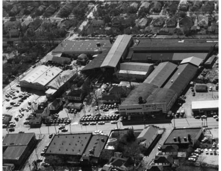
Aerial view of early 1960s expansion of the Stewart & Stevenson Harrisburg Plant
